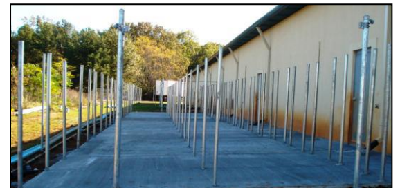
Construction is underway on the new kennel runs.
